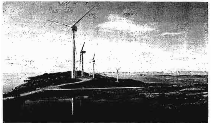
General Electric’s ScanWind offshore technology wind turbines.
