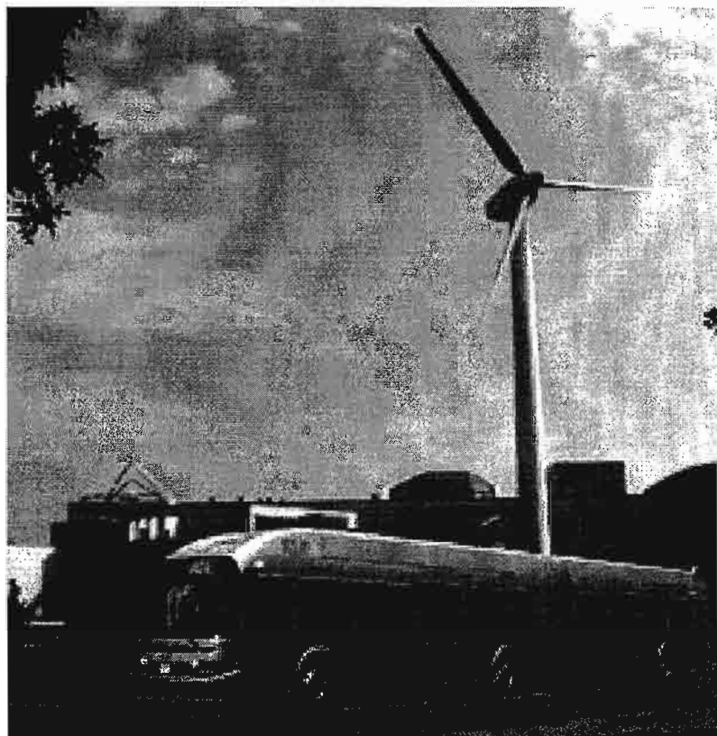
NASA's Glenn Research Center is designing a wind/sun-powered fueling system with zero carbon emissions for specially equipped city buses. An electrolyzer splits water molecules into oxygen and hydrogen, to be used for fuel cell-powered vehicles. Photo NASA/RTA.
