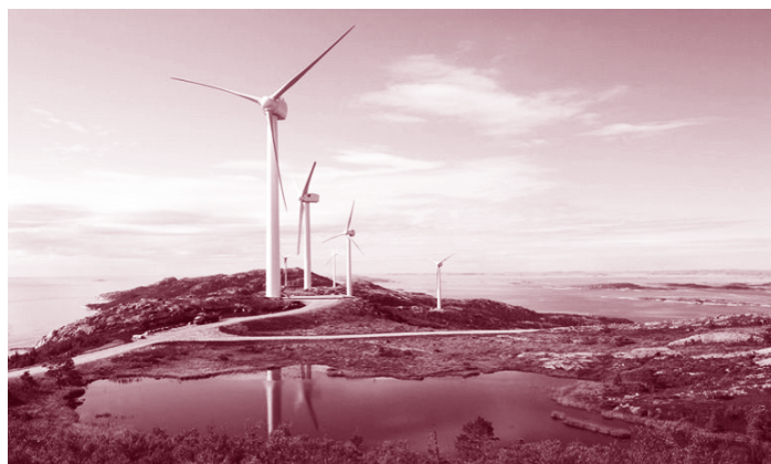
General Electric’s ScanWind offshore technology wind turbines.
